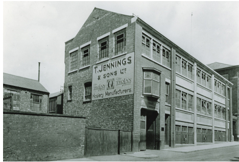
Plate 10a. Timothy Jennings & Sons Ltd The factory was built in the late 1920s. The building where he set up in business can be seen in the background. (The Earl Shilton and Barwell Photographic Archive)
